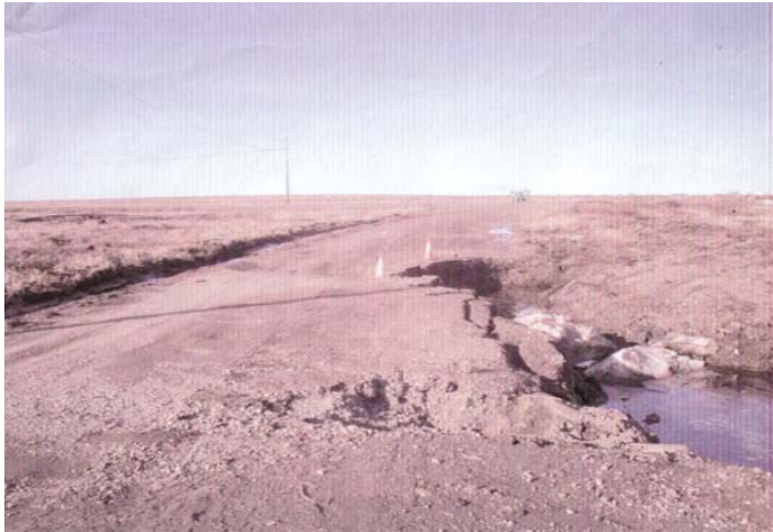
Photo 1: Erosion of road at the airport caused by Innachuk River, No photo date available.
