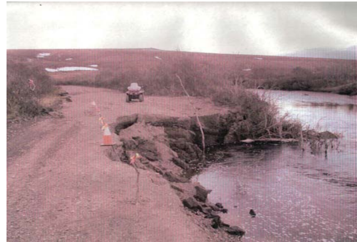
Photo 2: Erosion on road past airport, No photo date available.
